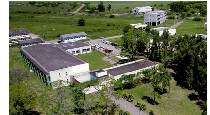
Campus Dom Pedrito
